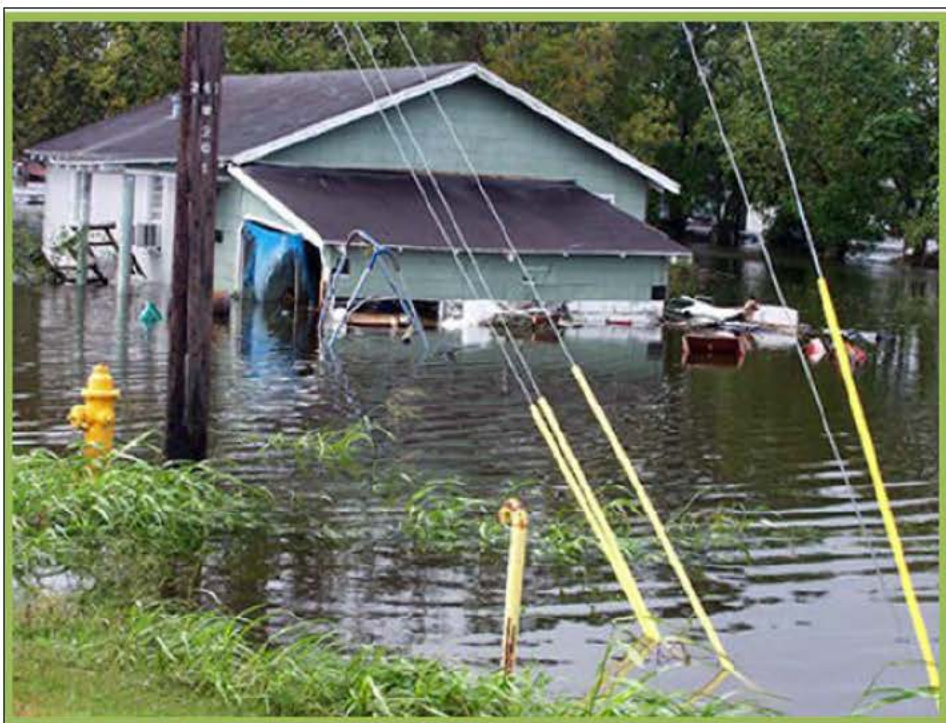
Hurricane Ike flooding in Delcambre, Louisiana 2008.
